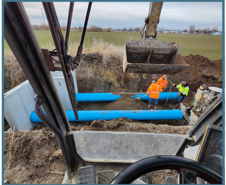
Maintenance crew replaces headgate 415-2, Photo credit: Wayne Sherbeck, January 2026
