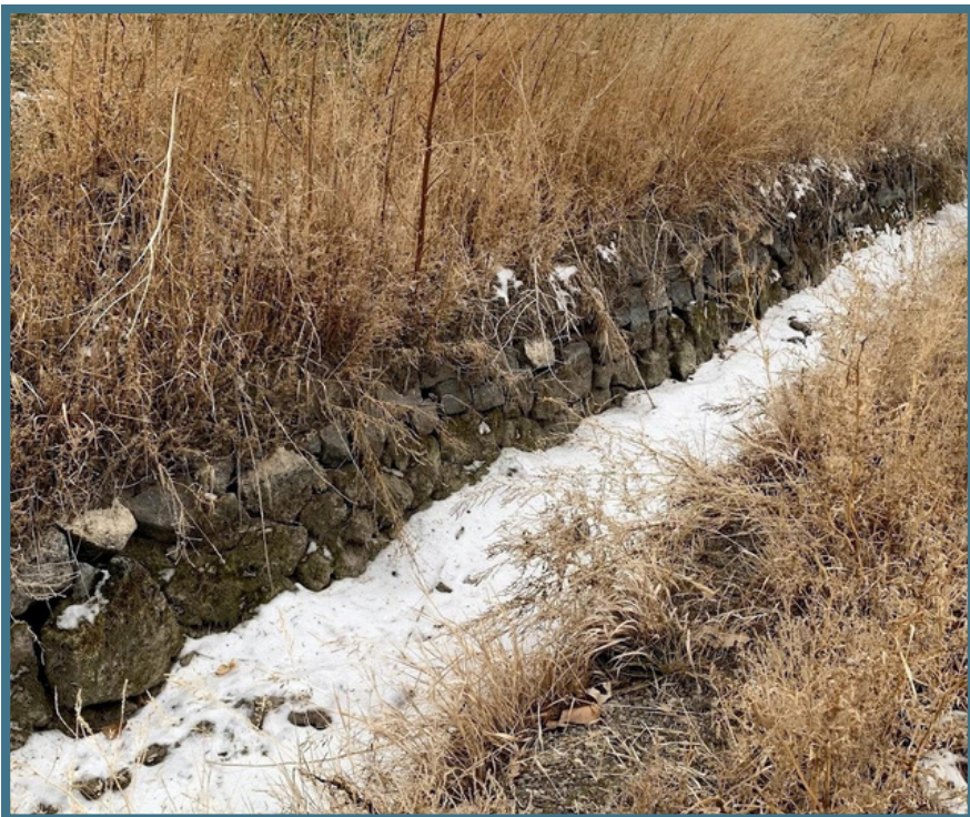
Lateral 39's rock lined channel prior to piping
