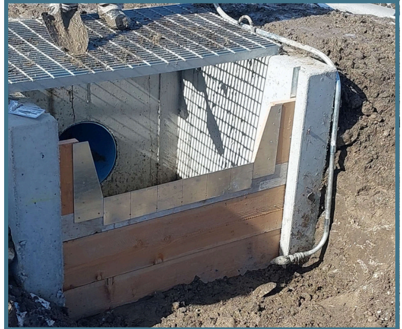
Lateral 33 Spill weir and automation installation Photo credit: Brandon Clement, February 2024
