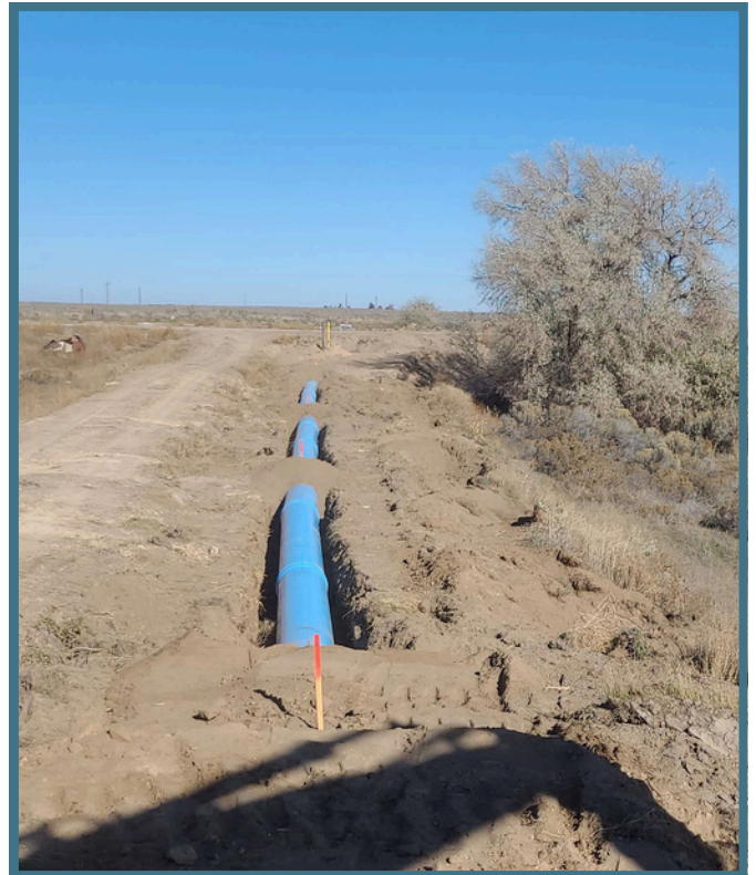
Newly installed pipe at Lateral 24 Photo credit : Evan Overson, November 2023
