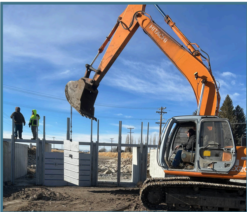
MID crews install new gates on the B2 Check Structure
